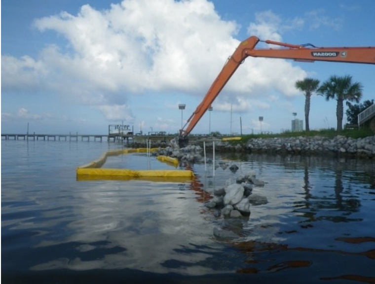
FIGURE 5: PHASE 1 CONSTRUCTION OF THE BREAKWATER
