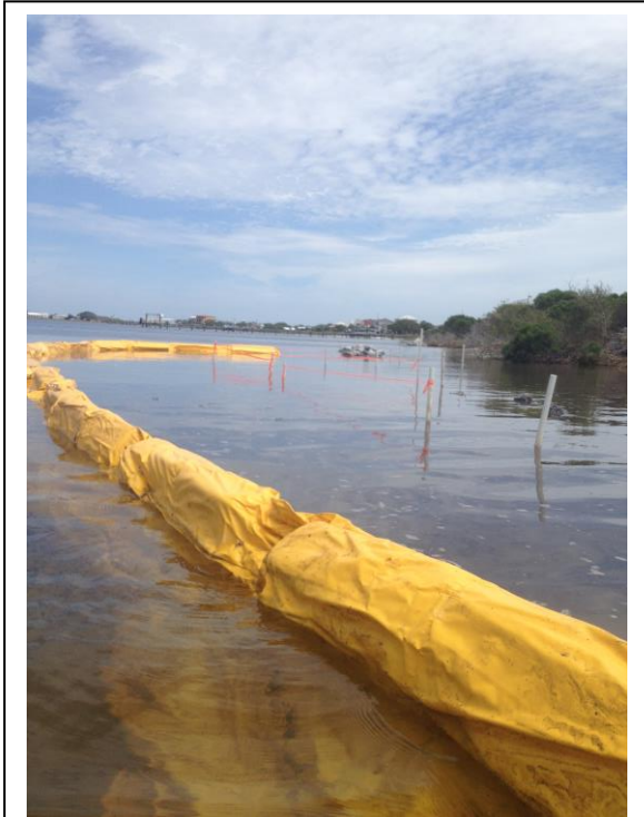
Fig. 10 -Curtain to protect seagrass and water quality
