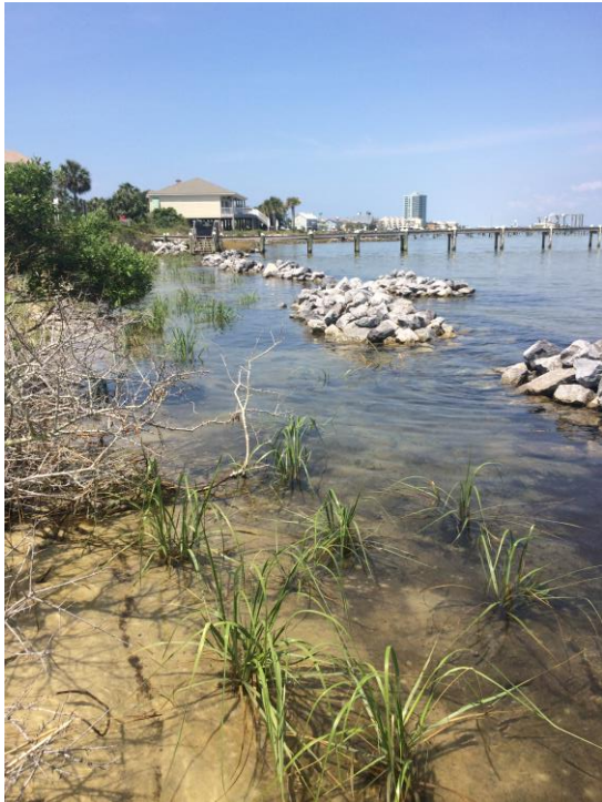
Fig. 33 Mid section left at sea level to flush into wet area
