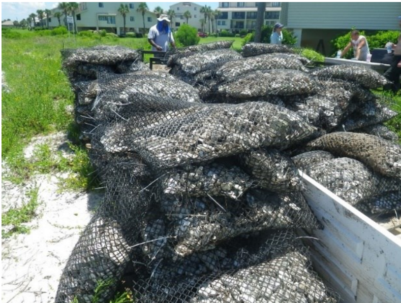
FIGURE 4: PHASE 1 PURCHASED OYSTER SHELL LOADED INTO MESH BAGS
