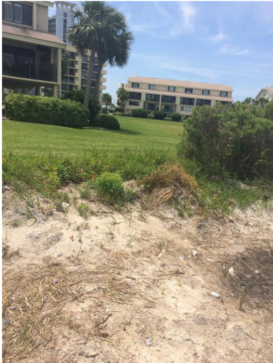
Fig. 29 -Spreading out sand to determine the elevation for the appropriate plants
