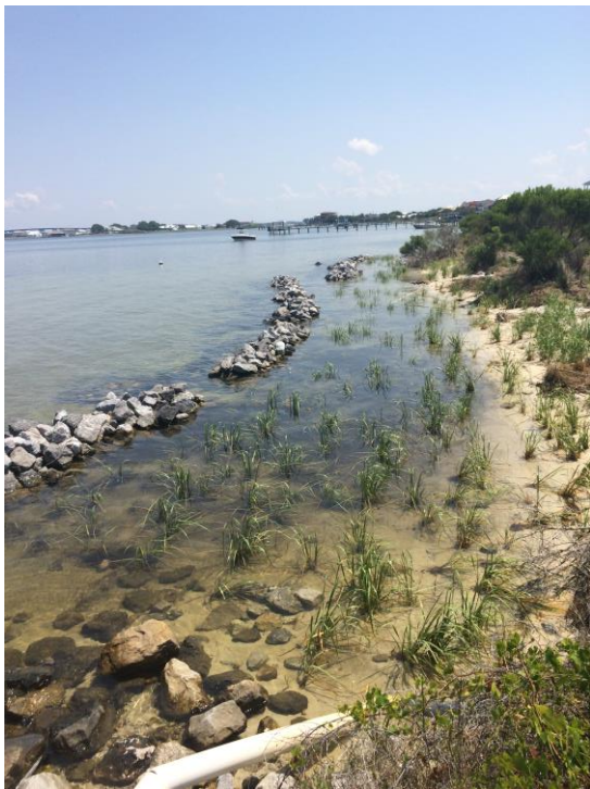
Fig. 35-Finished project left to establish
