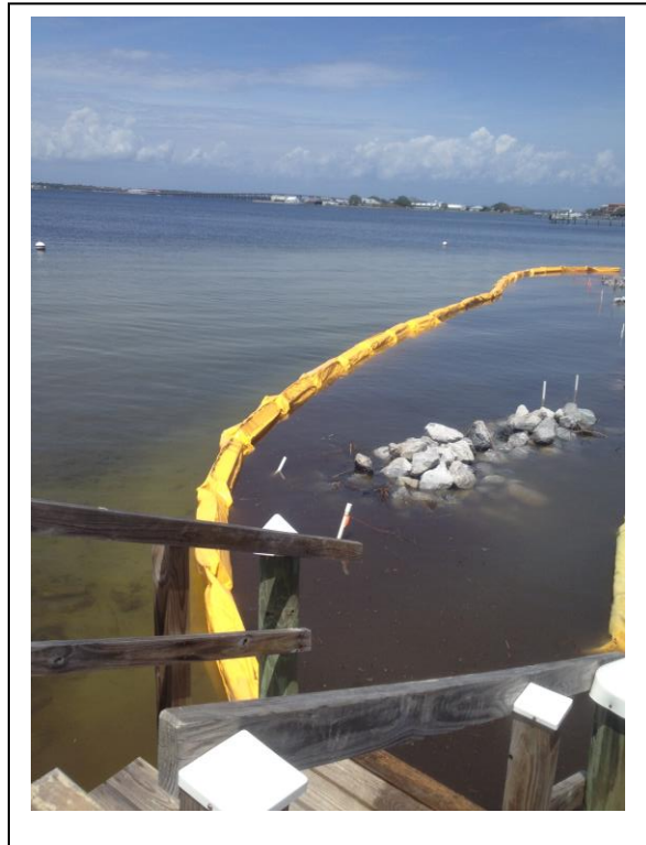
Fig. 16- The turbidity curtain containing the silt and sediment
