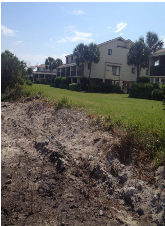
Fig. 23 Area containing rip rap- this area was replanted
