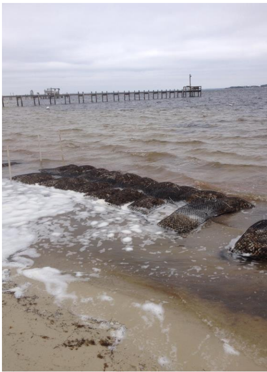
Fig. 25- Setting up oyster reef foundation
