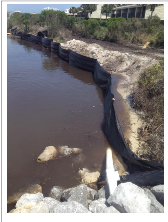
Fig. 15 -Berming of the side to create a slope to protect the property
