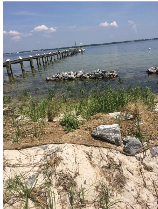
Fig. 36- Meshed mat used to provide additional stabilization to the shoreline
