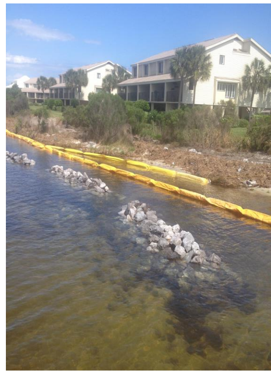
Fig. 26- Riprap placement over the oyster reef foundation
