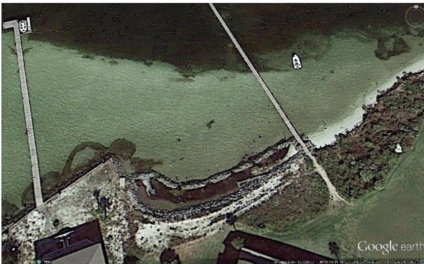
FIGURE 7: AERIAL OF COMPLETION OF PHASE 1
